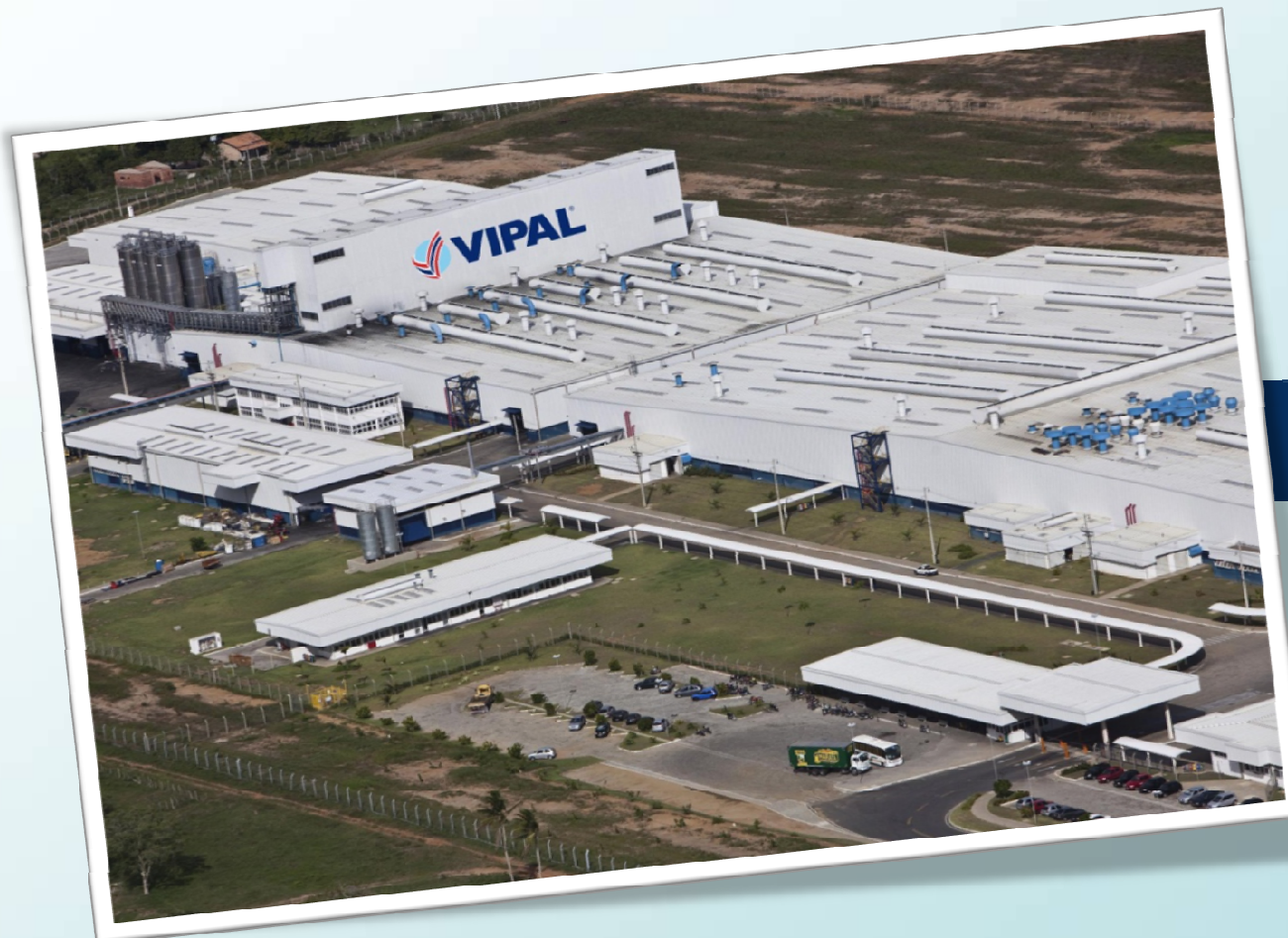
Fábrica 3 Borrachas Vipal
